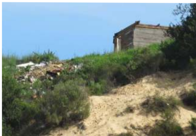
An informal structure - though not a new one - peeks over the top of the dune. The large pile of rubbish to its left is angering residents living in the areas below the dune.
