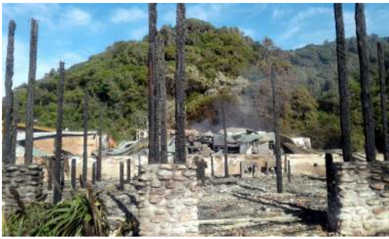
Fire completely guts Storms River Cattle Baron Restaurant & Shop
